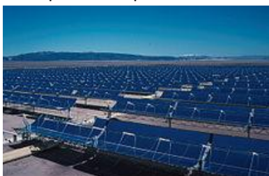
The 354 MW SEGS solar complex in San Bernardino, California USA.
