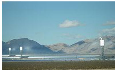
Ivanpah solar plant in the Mojave Desert, California , USA.
