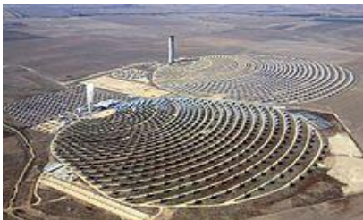
Solar Towers of the PS10 and PS20 solar plants in Spain.
