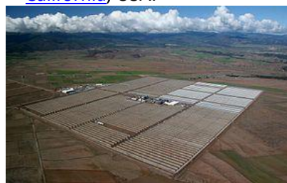
The 150 MW Andasol Solar Power, Station in Andalusia, Spain
